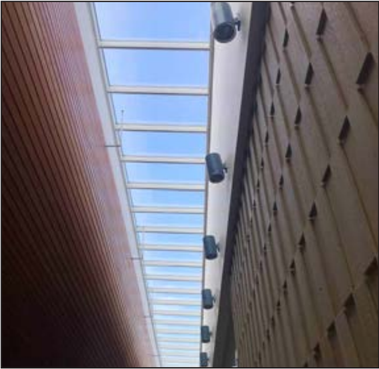
contributed photo Newly installed glass skylights in the main hall.
